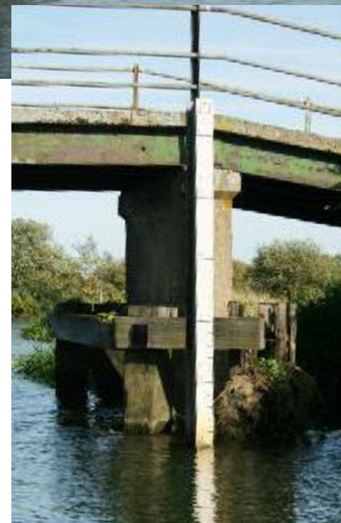
Gauge boards at bridges (below) let you know if you'll pass underneath
